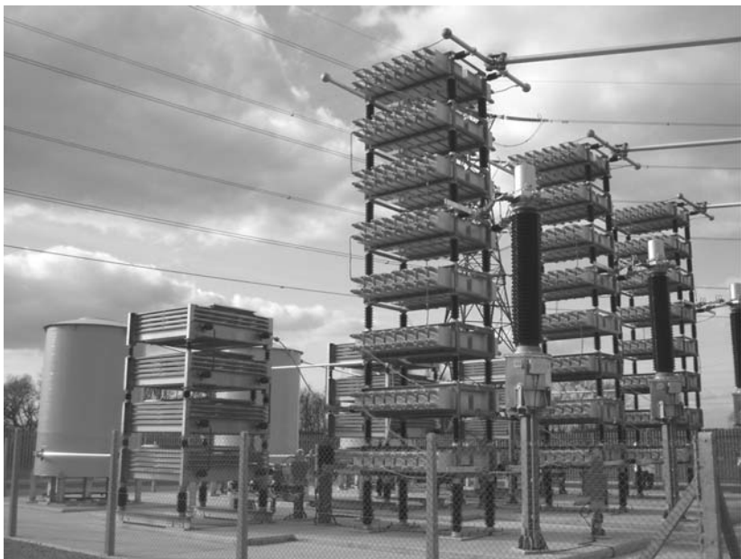
Figure 4.43 (a) 60 MVar 132 kV Mechanically Switched Capacitor (MSC) and (b) 400 kV 225 MVar MSC (with an RLC damping network)
