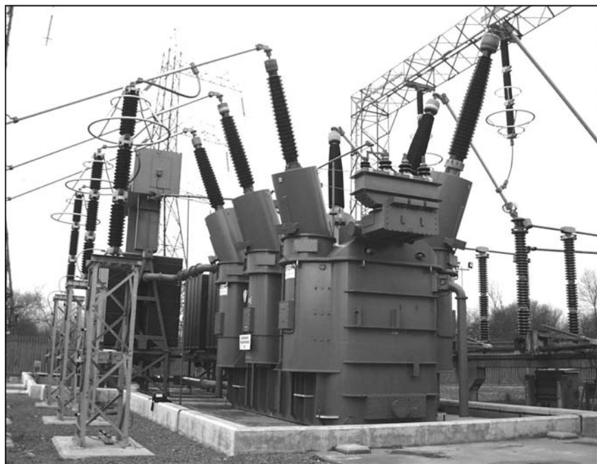
Figure 4.2 1000 MVA 400 kV/275 kV autotransformer
