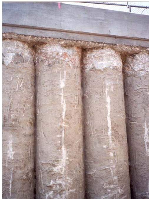
Figure 5-8 Tangent Pile Wall Construction Schematic
