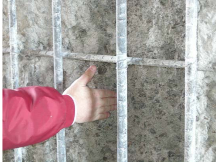
Figure 16-7 Substrate after Hydro-demolition, Shawmut Jct. Boston
