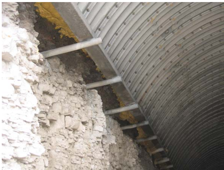
Figure 16-20 Rock Bolts (Dowels) Supporting Liner, I-75 Lima Ohio Underpass
