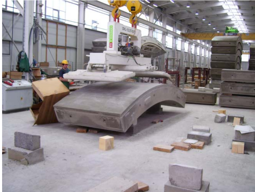
Figure 10-7 Precast Segments for One-Pass Lining, Forms Stripped
