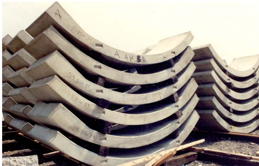
Figure 10-9 Stacked Precast Segments for Two-Pass Lining
