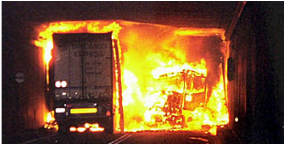
Figure 1-11 Gotthard Tunnel Fire in October 2001 (FHWA 2006)
