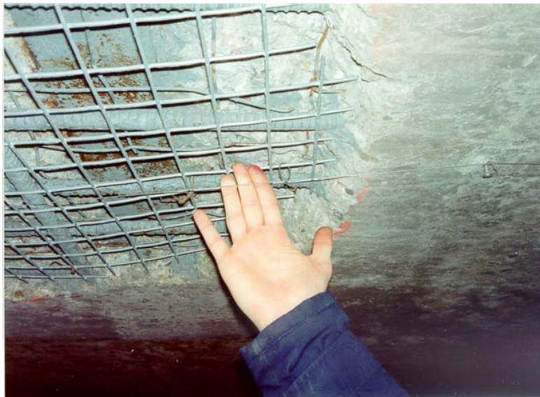
Figure 16-12 Reinforcing Steel for Repair, Sumner Tunnel Boston
