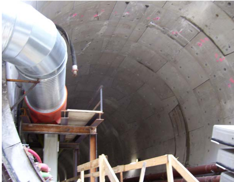
Figure 10-2 Precast Segmental Lining
