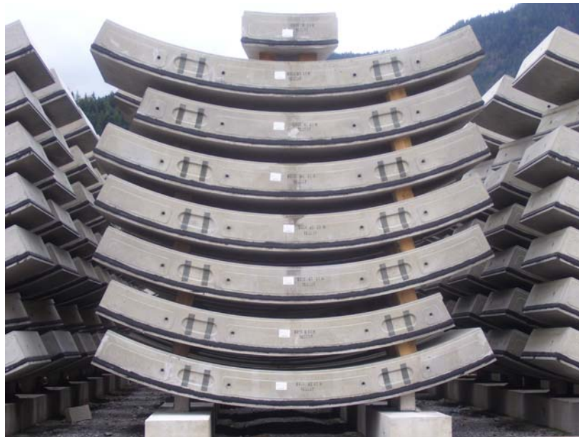
Figure 10-8 Stacked Precast Segments for One-Pass Lining
