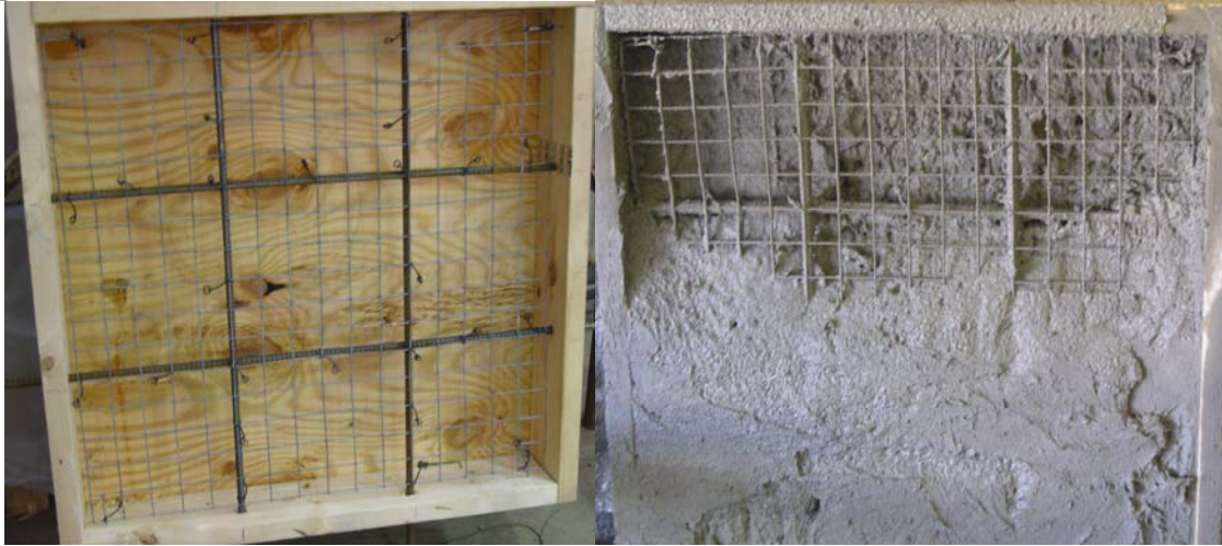
Figure 16-16 Cast Iron Segmental Segment Mock-up of Filling with Shotcrete, MBTA Boston
