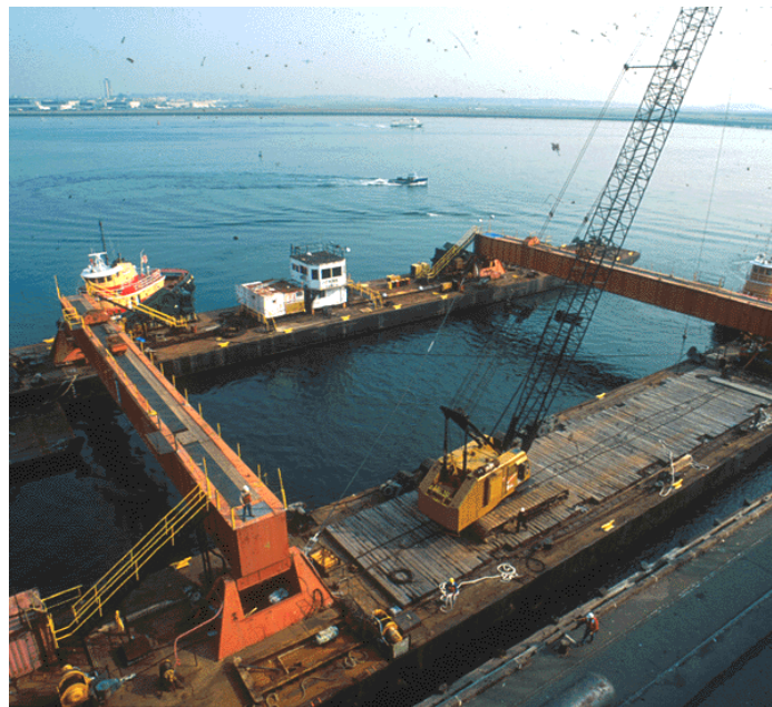
Figure 11-14 Catamaran Lay Barge
