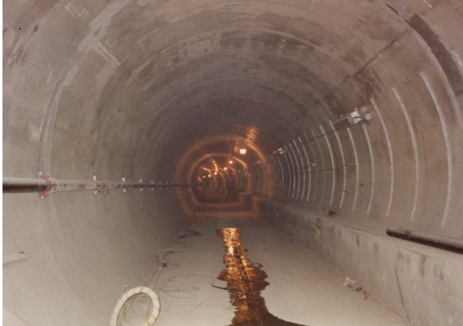
Figure 10-6 Cast-In-Place Concrete Lining, Washington DC
