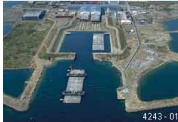
Figure 11-10 Fabrication Facility and Transfer Basin, Øresund Tunnel, Denmark
