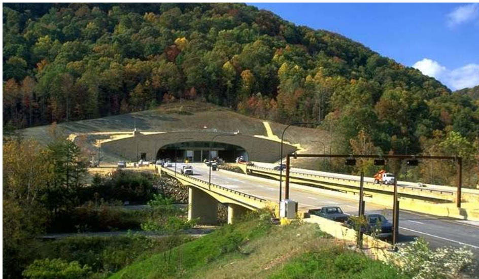
Figure 2-8 Portal Structure for Cumberland Gap Tunnel
