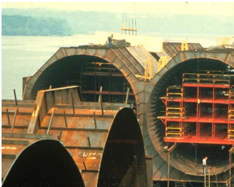
Figure 11-6 Fort McHenry Tunnel, Baltimore
