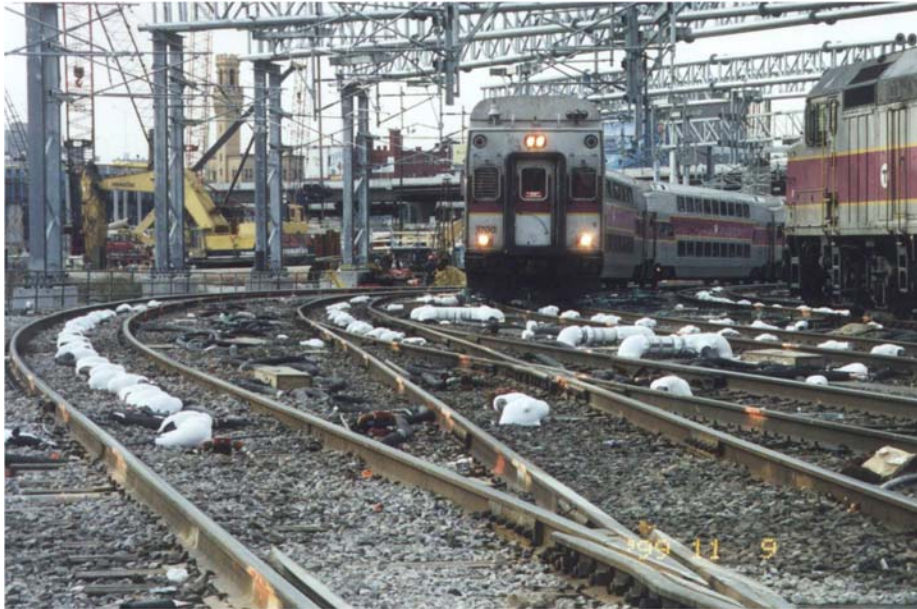
Figure 12-12 Ground Freezing System in Operation while Commuter Trains Run Through the Area
