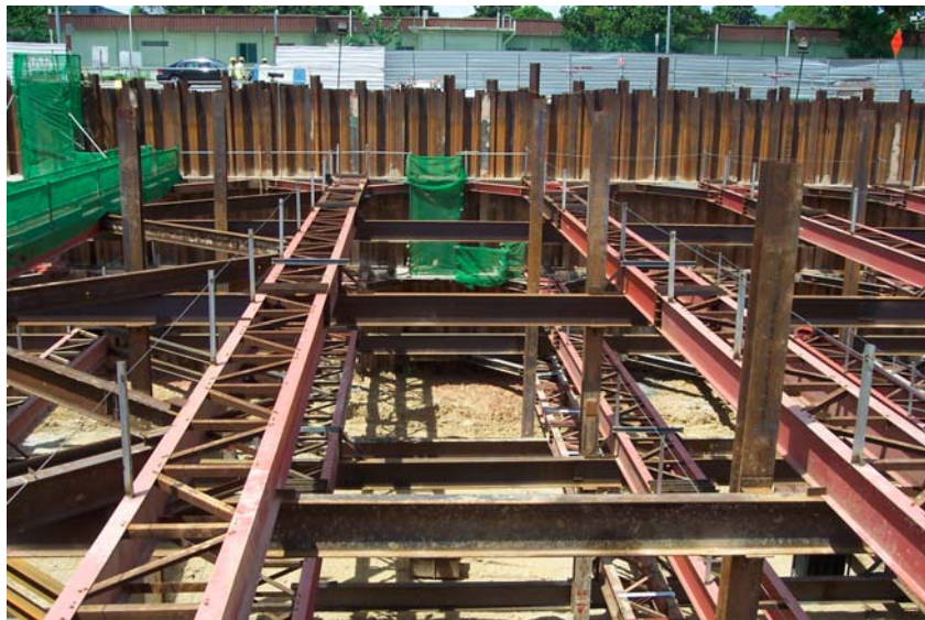
Figure 5-4 Sheet Pile Walls with Multi Level-Bracing
