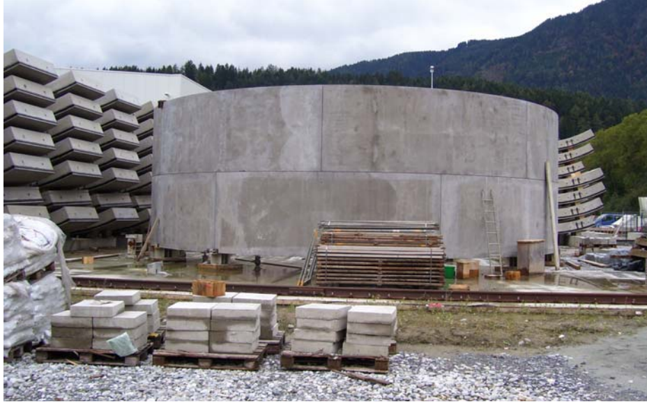
Figure 10-13 Mock-up of Precast Segment Rings
