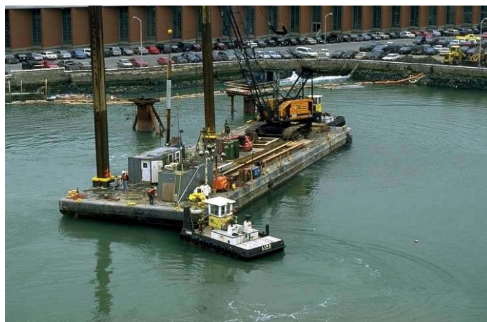
Figure 11-9 Fort Point Channel Tunnel, Boston
