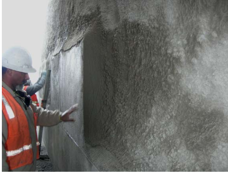
Figure 16-13 Shotcrete Finishing, Shawmut Jct. Boston
