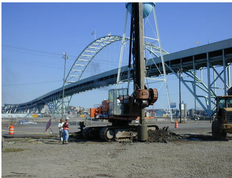
Figure 3-7 Rotosonic Sampling for a CSO Tunnel Project at Portland, Oregon.
