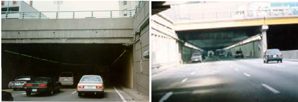
Figure 2-7 “Black Hole” (Left) and Proper Lighting (Right)
