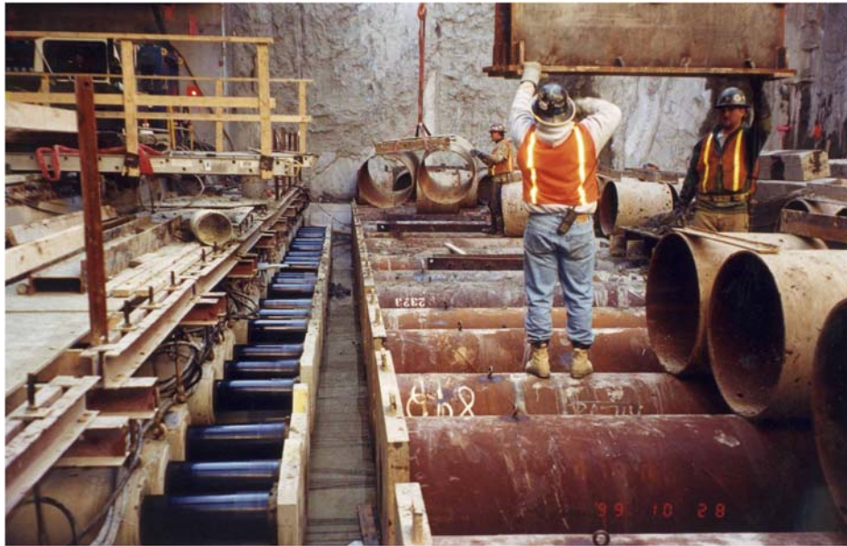
Figure 12-8 Installation of Packer Sections and Connecting Diaphragm Plates
