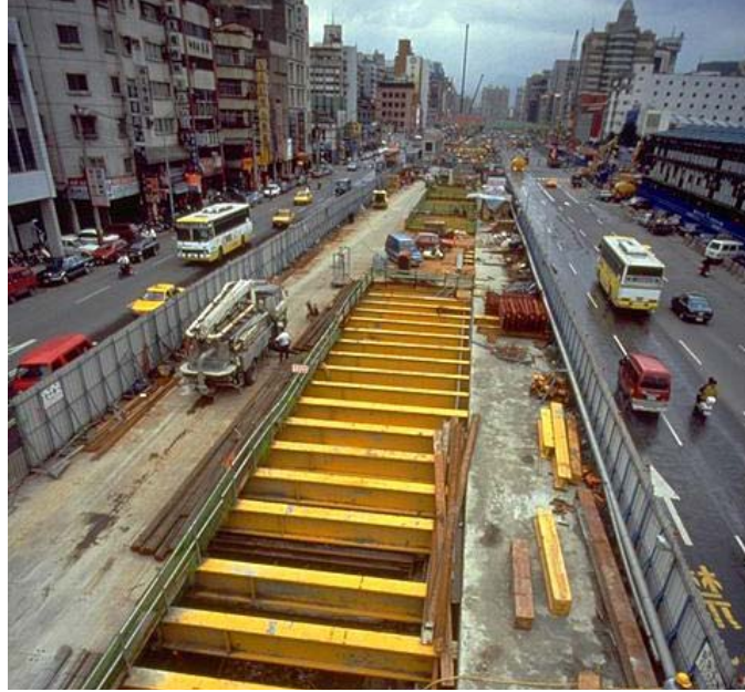
Figure 5-7 Braced Slurry Walls
