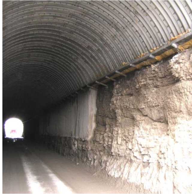
Figure 16-19 Rock Tunnel with Shotcrete Wall Repair and Arch Liner (I-75 Lima Ohio)
