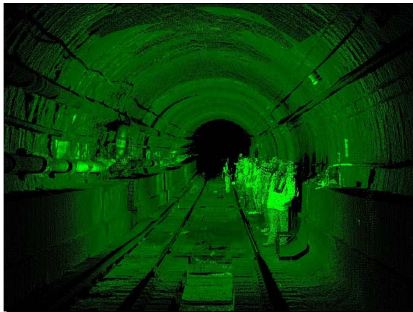
Figure 3-3 3D Laser Scanning Tunnel Survey Results in Actual Scanned Points
