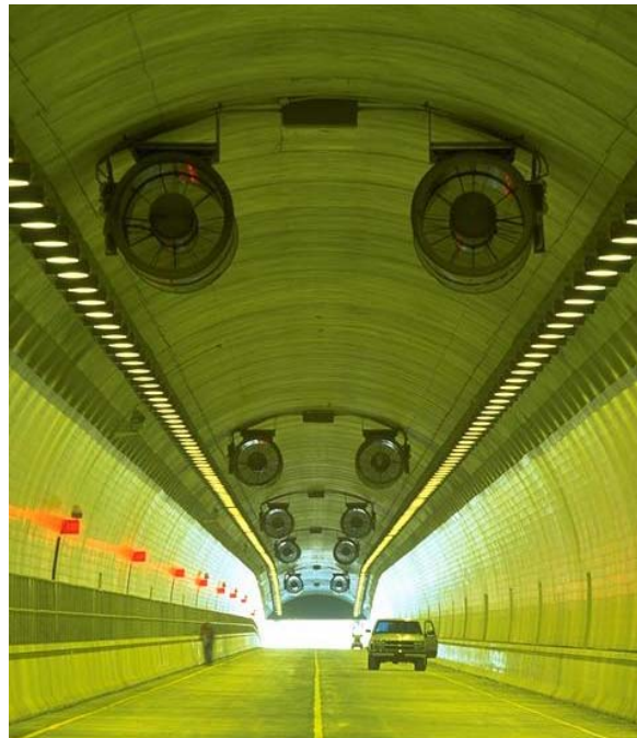
Figure 10-1 Cumberland Gap Tunnel
