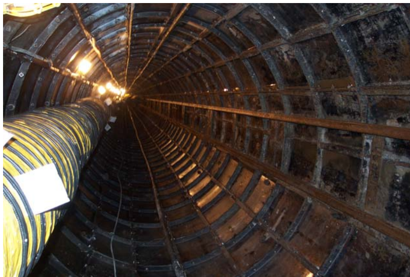
Figure 10-3 Baltimore Metro Steel Plate Lining
