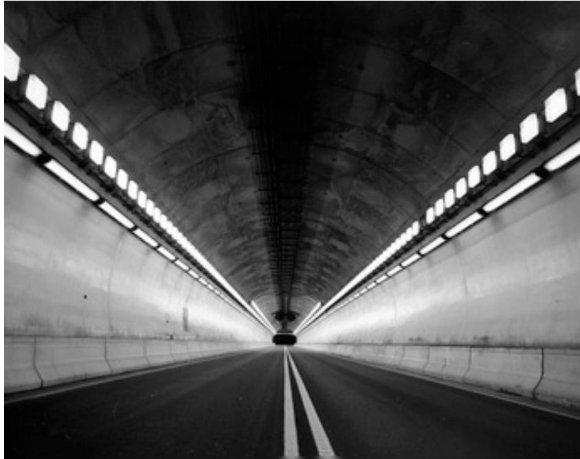
Figure 10-4 New Lehigh Tunnel on Pennsylvania Turnpike Constructed with Final Shotcrete Lining
