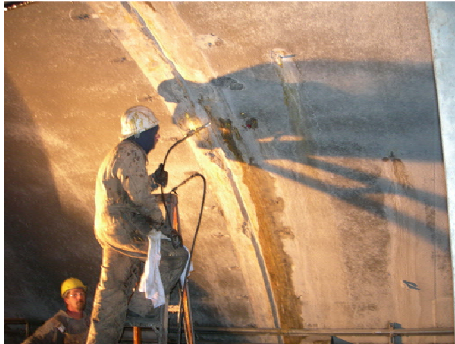
Figure 16-4 Leak Injection, Tuscarora Tunnel PA Turnpike
