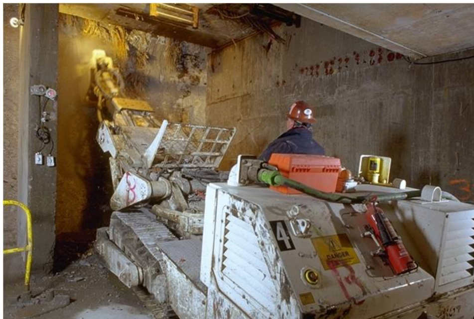
Figure 12-5 Excavation of the Frozen Ground at the Front of the Tunnel Shield by Roadheader
